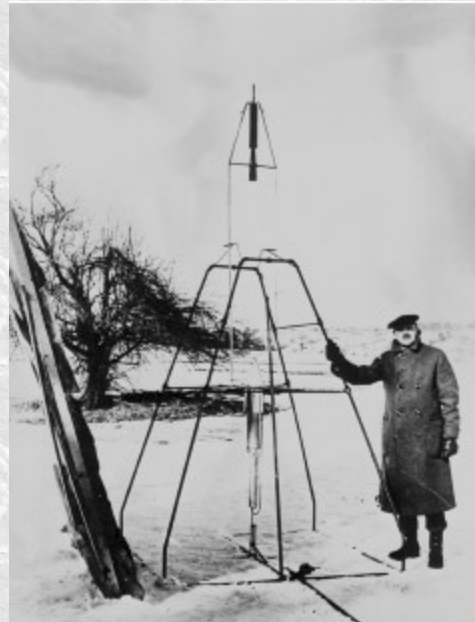
Dr. Robert H. Goddard and His Rockets: Dr. Goddard and liquid oxygen-gasoline rocket in the frame from which it was fired on March 16, 1926, at Auburn, Massachusetts. It flew for only 2.5 seconds, climbed 41 feet, and landed 184 feet away in a cabbage patch. From 1930 to 1941, Dr. Goddard made substantial progress in the development of progressively larger rockets, which attained altitudes of 7800 feet. Credit: NASA
